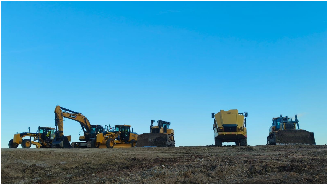
Figure 2 – Construction Equipment on Site
